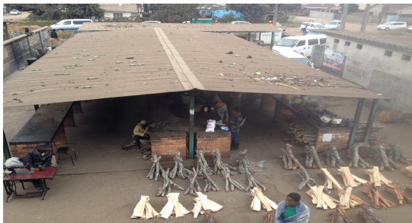
Plate 1: Gazaland market in a dilapidating state.
